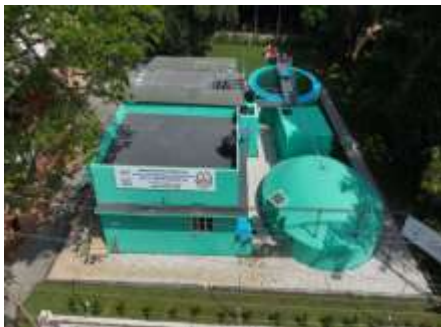
360 KLD STP at General Hospital, Thrissur
