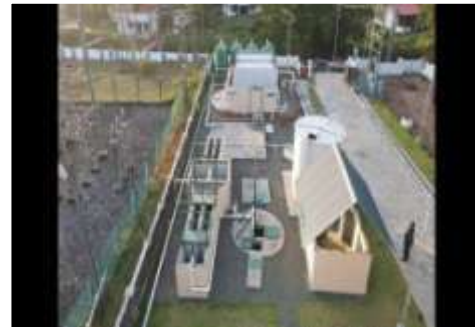
1 MLD CSTP at Padanappalam, Kannur
